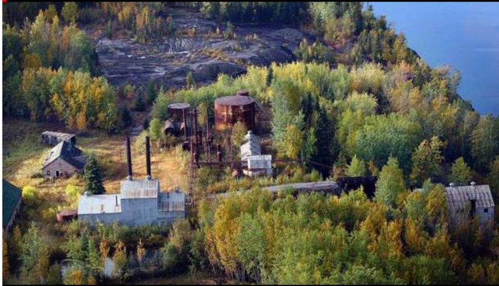
1929: After field tests in 1924, scientist Karl Clark and associate Sidney Blair patent their water-flotation system. 1930: Mr. Clark starts producing from a small plant at Bitumount, on the shore of the Athabasca River near Fort McMurray (shown here in 2011), pumping 300 barrels a day with a seven-man crew. The product is used largely for roofing and paving. (Jeff McIntosh/The Canadian Press)
