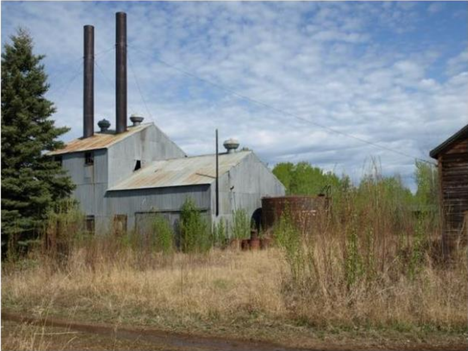
The powerhouse at Bitumount (photo by David Martin).
